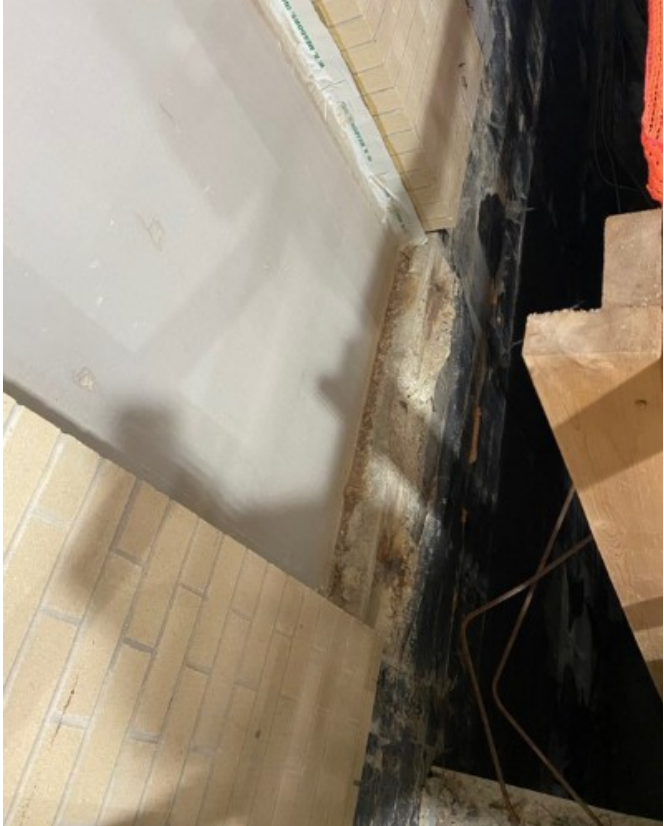
View of the tie-in gap between University Hospital and Children’s Hospital
